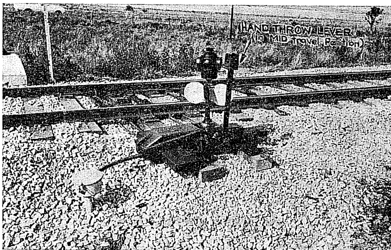
Diagram No. 2 G.R.S. Model 9 Hand Operated Switch Machine
